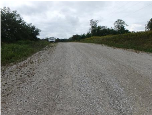
Photo 5: Existing Access Road Entrance
