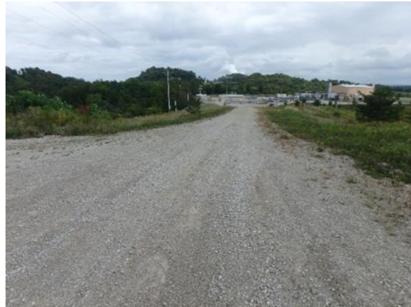
Photo 4: Existing Access Road traversing Project Area
