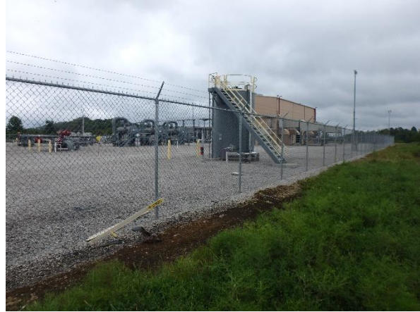
Photo 2: Existing Station Pad
