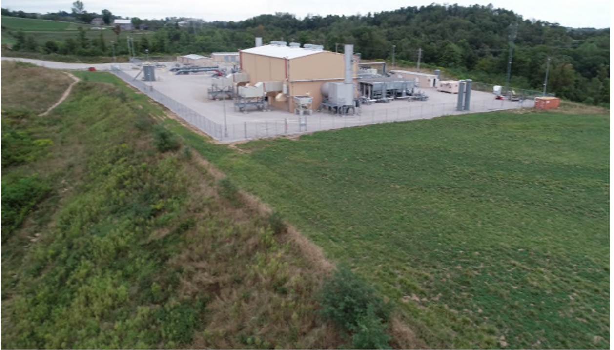
Plasma Compressor Station – Monroe County, Ohio
