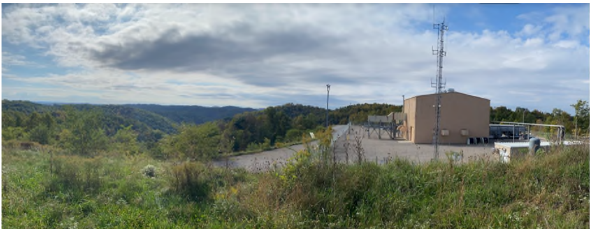
Corona Compressor Station – Wetzel County, West Virginia
